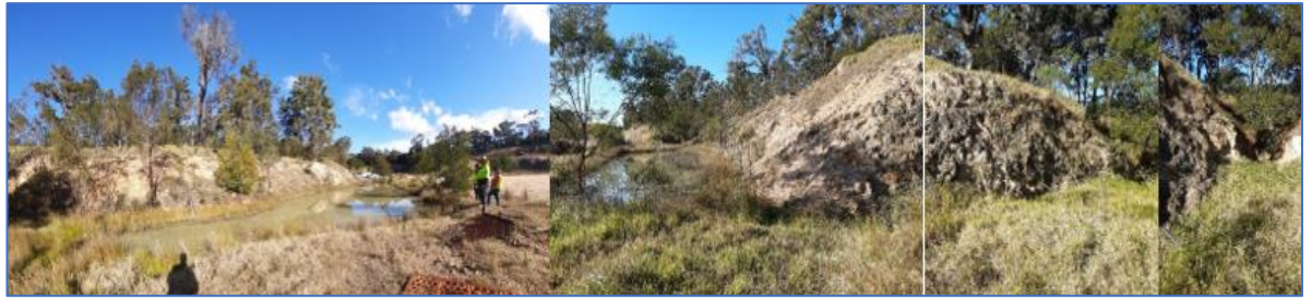
Photo 14 Perspectives of dam and drainage culvert onsite
