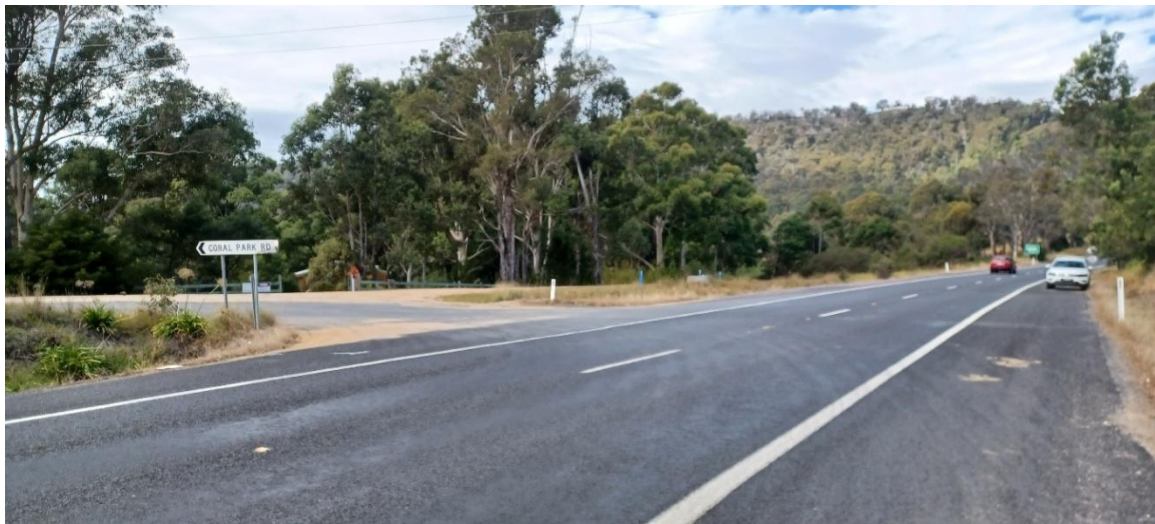
Figure 19 Princes Highway - Coral Park Road intersection facing south
