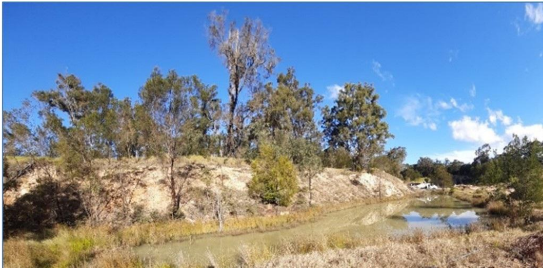
Photo 12 Existing Sedimentation Pond
