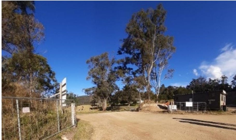
Photo 8 Quarry entrance from within the quarry site and site office
